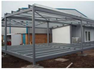
Top: Modular Cleanroom under construction
