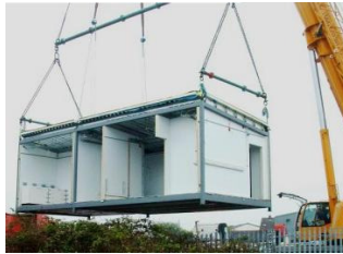
Bottom: Lifting a modular unit
